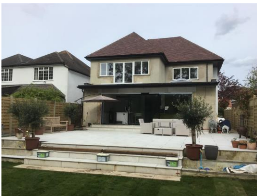
Figure: 7 Rear elevation April 2024
